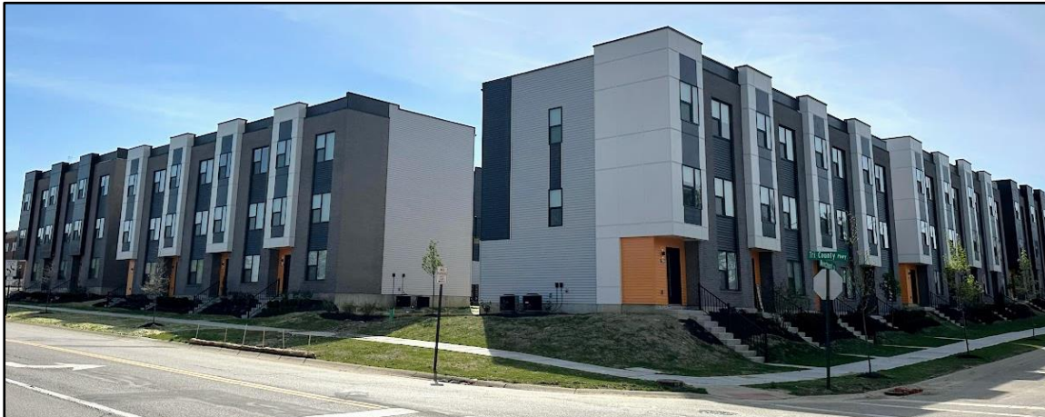
Row On Merchant Completed Townhomes (April 2023)
