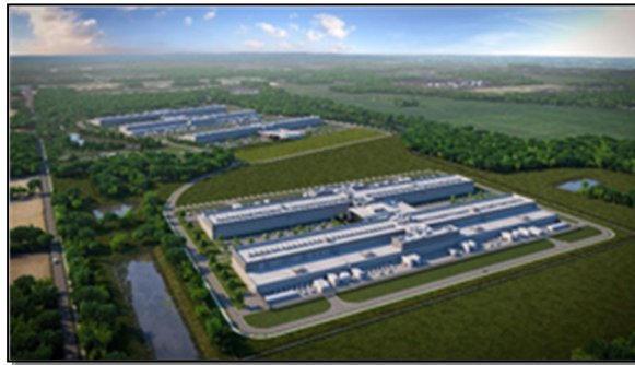
Figure 4 – Facebook New Albany Data Center
