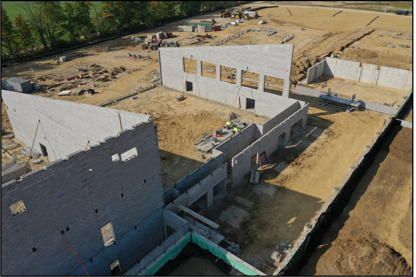
Berkshire K-12 Construction Site
