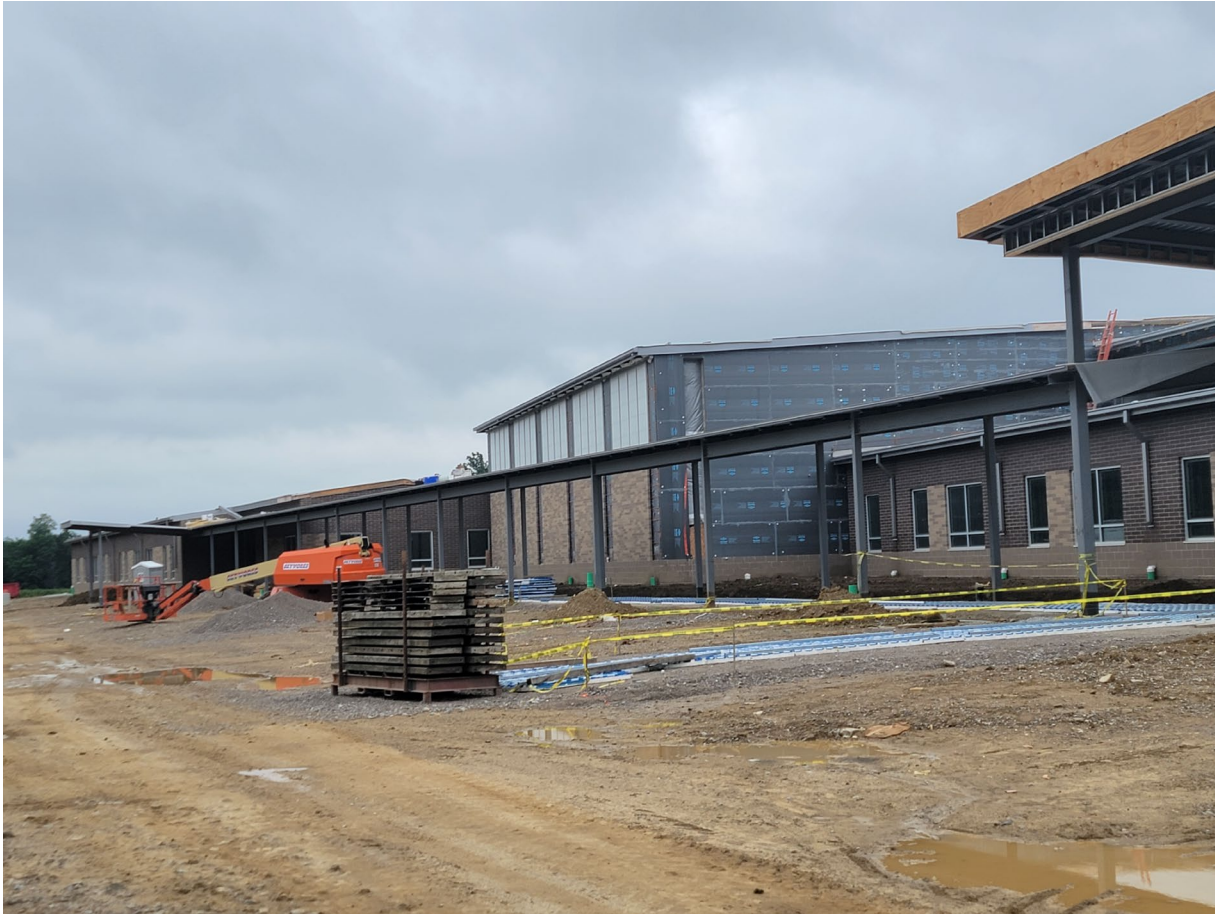
Berkshire K-12 Construction Site
