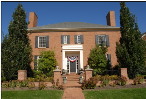
Figure 4 – Example of Residential Architecture
