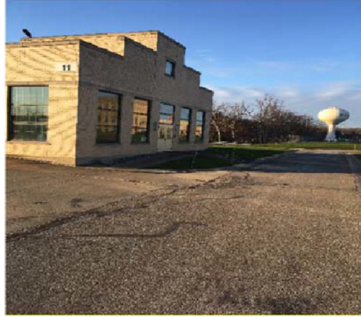
Photo 2: Photograph of the east side of the Carbon/Permanganate Building
