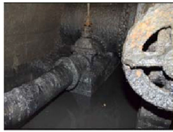
Photo 2: Existing valve proposed for replacement in the Phase IV Project.
