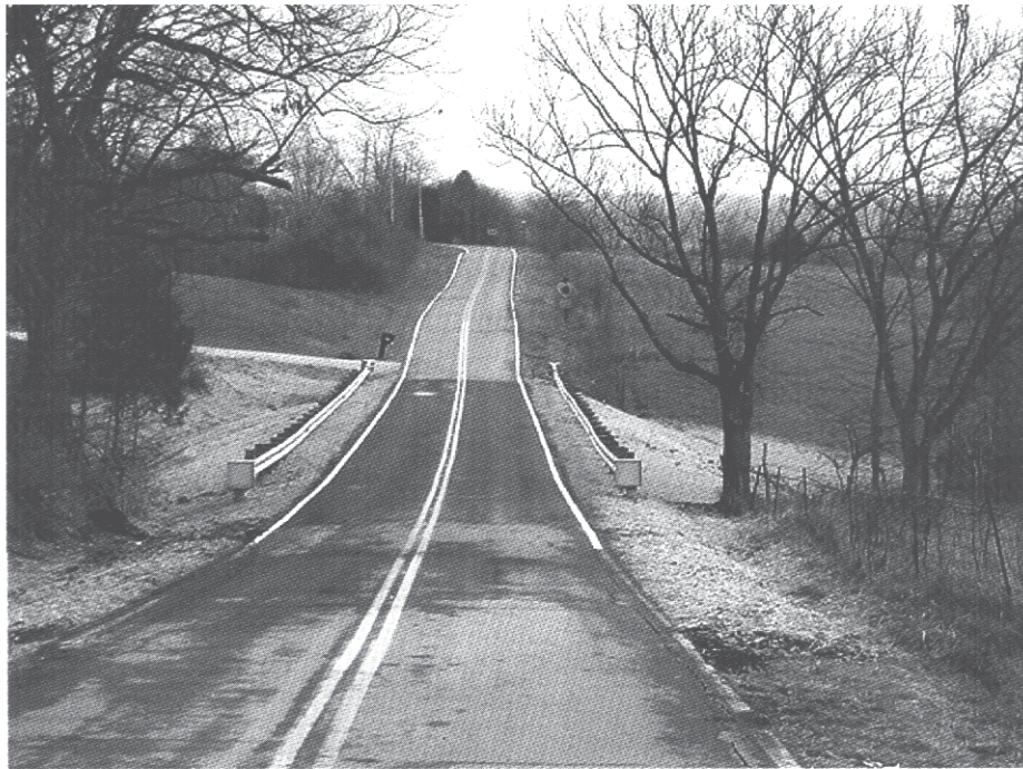
New bridge on Oxford-Middletown Road.
