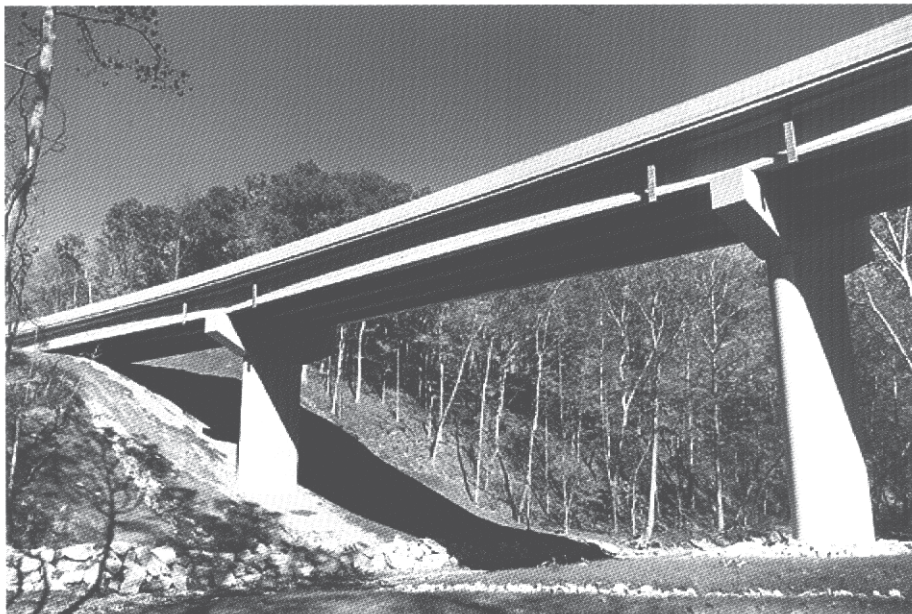
The new California Road Bridge over Dry Fork Creek constructed in 2002.
