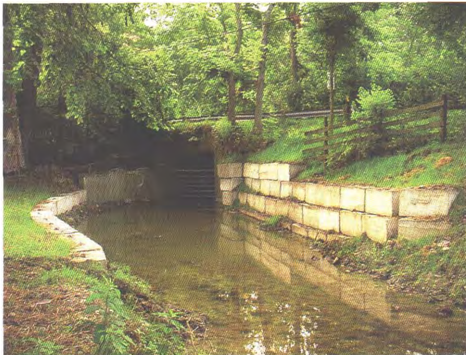
Four Mile Creek Bridge.
