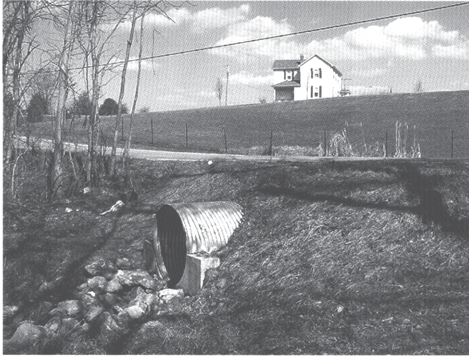
New Elk Creek Road Culvert.
