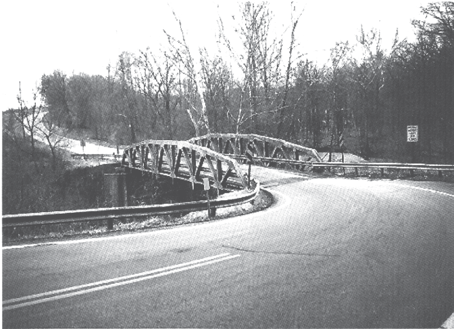
The old California Road Bridge constructed in 1953.
