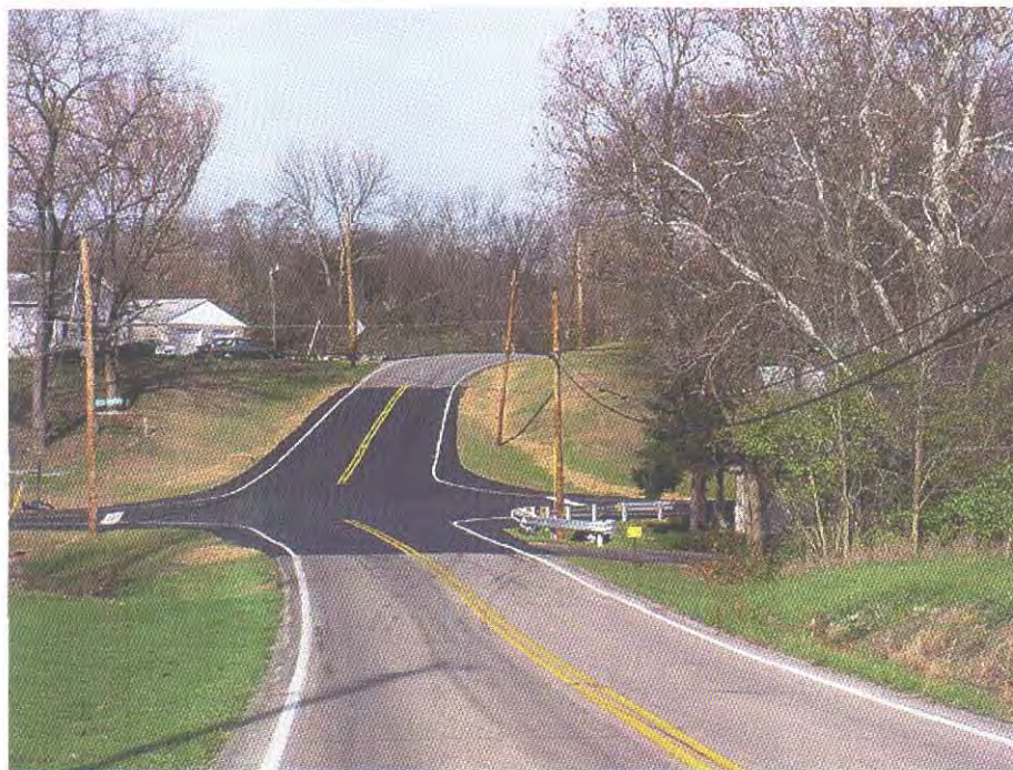
New intersection at West Alexandria Road and Elk Creek Road.
