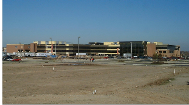
Reynolds and Reynolds — Phase II under construction
