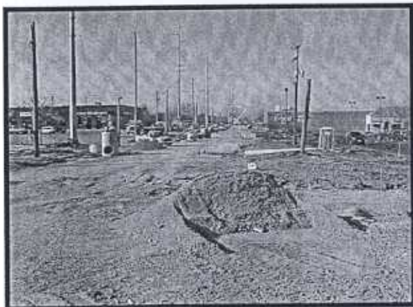
Hoover Road Reconstruction
